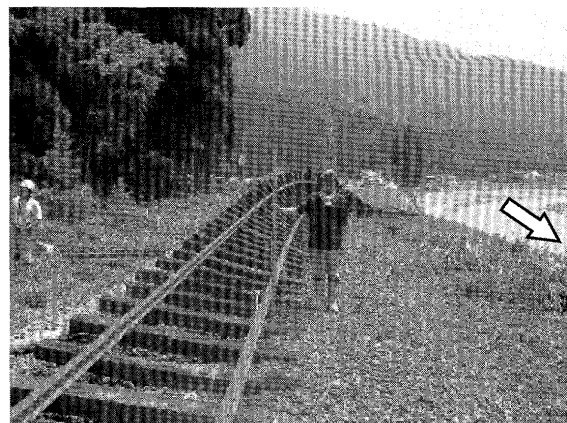
Photo 4. Rails and sleeper were moved toward the river due to the overflow at Shinagase in Miyama town
